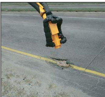
The hole is cleaned with a volume blower.
