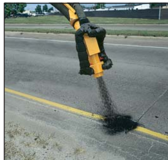
A tack coat of emulsion is applied to the area.
