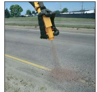
A finish coat of aggregate . . . and traffic flows.
