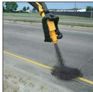
A mixture of aggregate and hot emulsion fills the hole.
